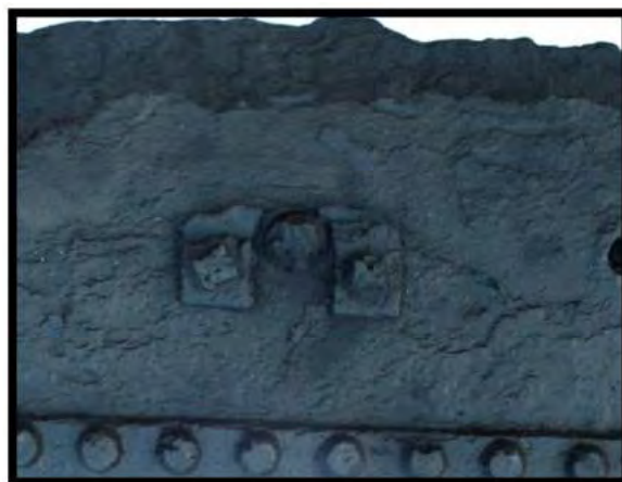
FIGURE 150. BROKEN TAB FOR SUPPORTING BEARING BARS (CLOSE UP SHOT FROM WATER LEG; ARTIFACT 132-001.79; ALSO SEEN IN FIGURE 136)
