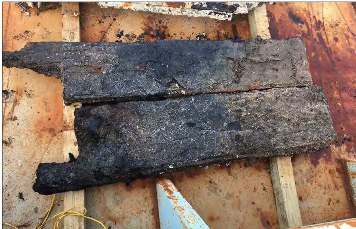
Figure 6-98. Lift WC-7. Originally one 4-foot wide piece, together they form a square, 27-inch wide, as-built cutout thought to represent a gun port. It will be found to be the only gunport on the entire length of the West Casemate.
