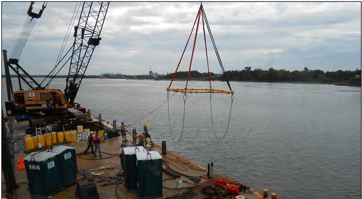
Figure 6-78. Rigging frame constructed that would hopefully allow for a successful second attempt at recovery of the casemate. This would not be the case.
