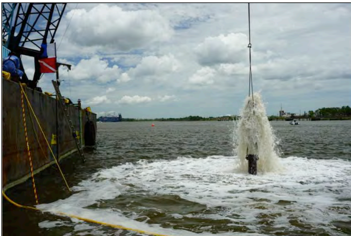
Figure 6-88. Airlift made of a 1-foot diameter 30-foot long iron pipe that was lowered into place by crane and then positioned by diver prior to beginning airlifting on both the East and West Casemates.
