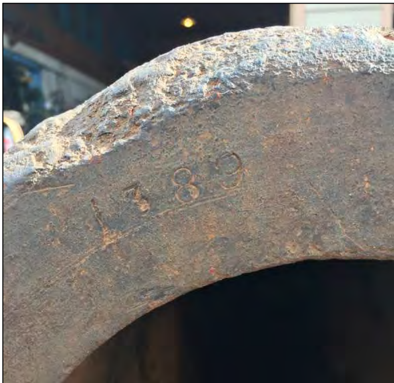
Figure 6-285. IX-Inch Dahlgren, Cannon No. 2, Artifact 1612, the breech stamped with “1389,” which is the foundry number.
