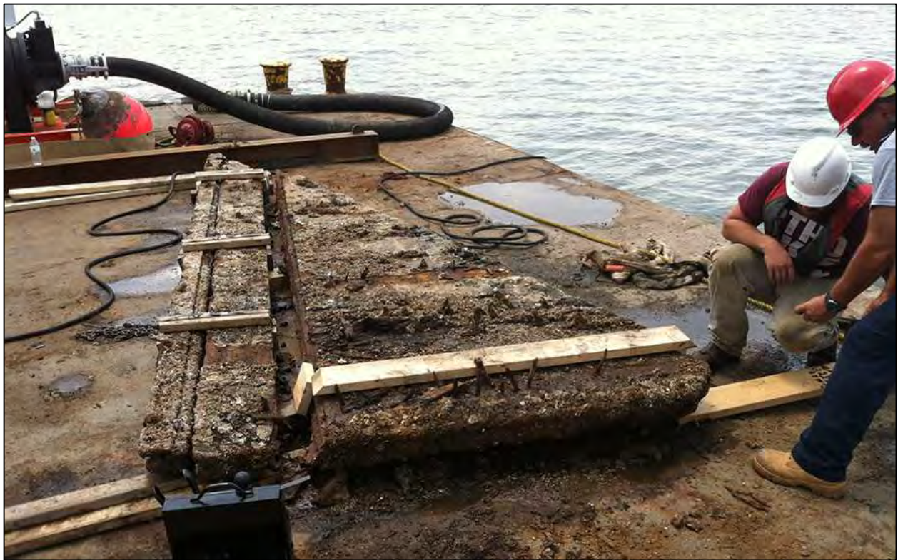
Figure 6-69. Northern, triangularly shaped, first section recovered (No. 1) being readied for shipment. Note the lack of wood backing on the inner face, as evidenced by the spikes that would have attached the wood being visible.
