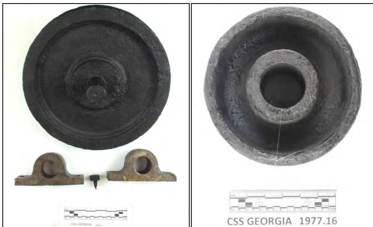
Figure 6-345. Pivot carriage truck and small copper-alloy journals recovered from Unit 7-F (Artifact 2934.01, left) compared to a top carriage truck recovered from Unit 7-A (Artifact 1977.16, right).
