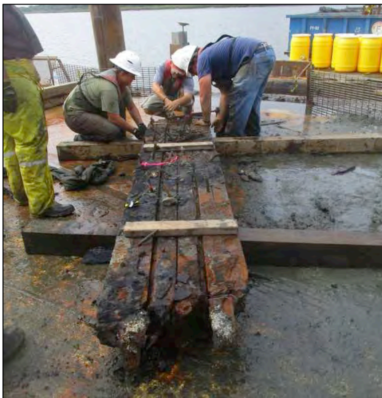
Figure 6-62. Bundling rails on the South Casemate. The angle of the side can be seen on the near end.
