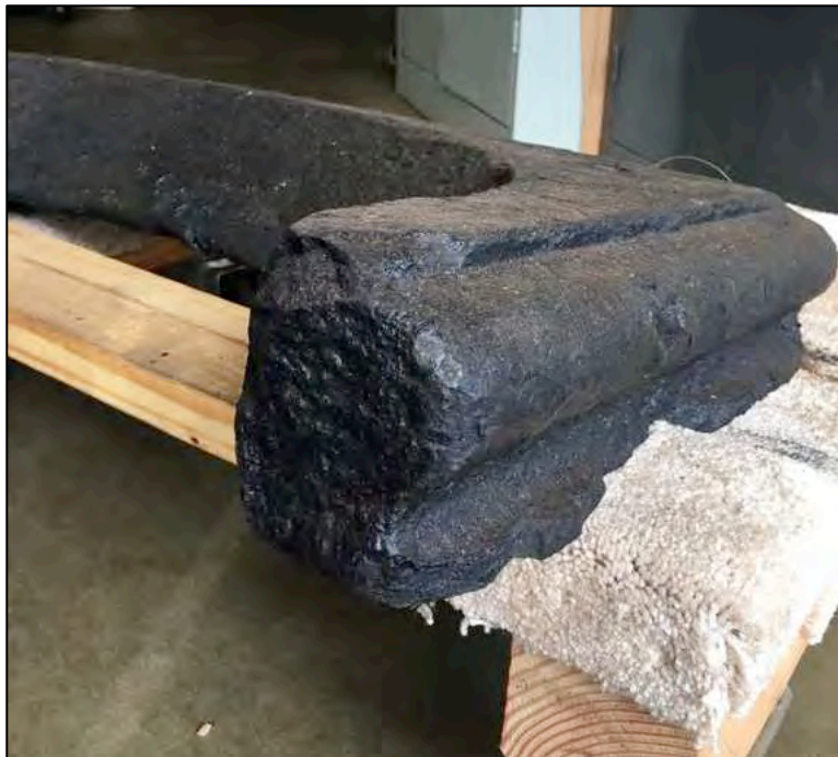
Figure 6-527. Artifact 2049, the gunport sides were cast in the shape of a half section of rail to accommodate overlapping and interlocking attachment with adjacent rails on the casemate.
