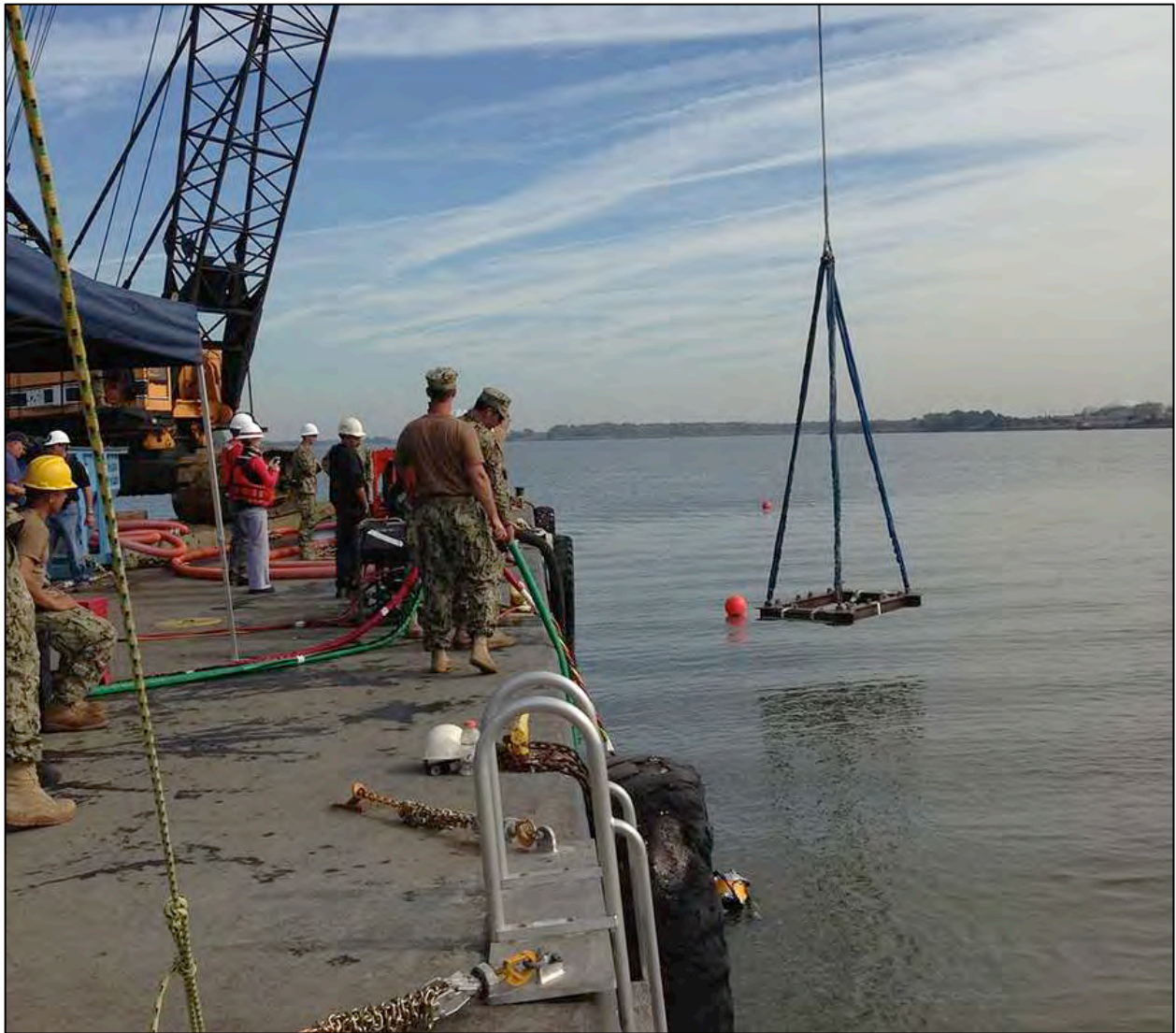
Figure 3-16. Iron I-beam cradle being lowered down to the recovery section.
