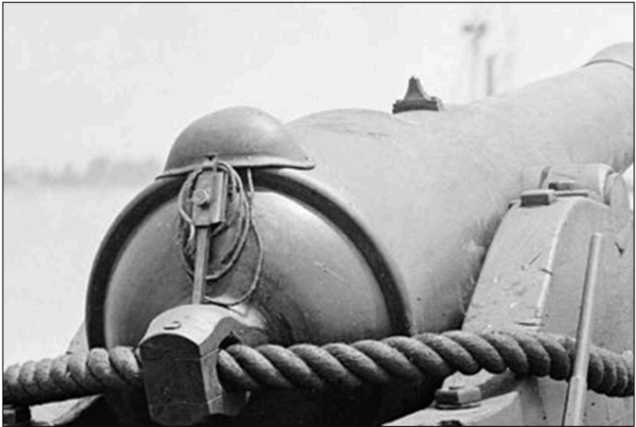
Figure 6-312. Brooke Rifle on the CSS Teaser showing the location of the tangent sight above the cascabel, and dispart sight forward in the center of the gun. Note the percussion lanyard placed around the tangent sight and that runs under the percussion lock cover for firing (as presented in Miller and Lanier 1911:77).
