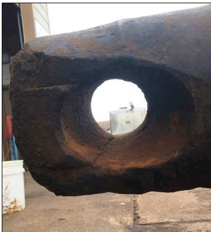
Figure 6-288. View of cascabel showing it is a composite or has an insert completing the circular opening for rope.
