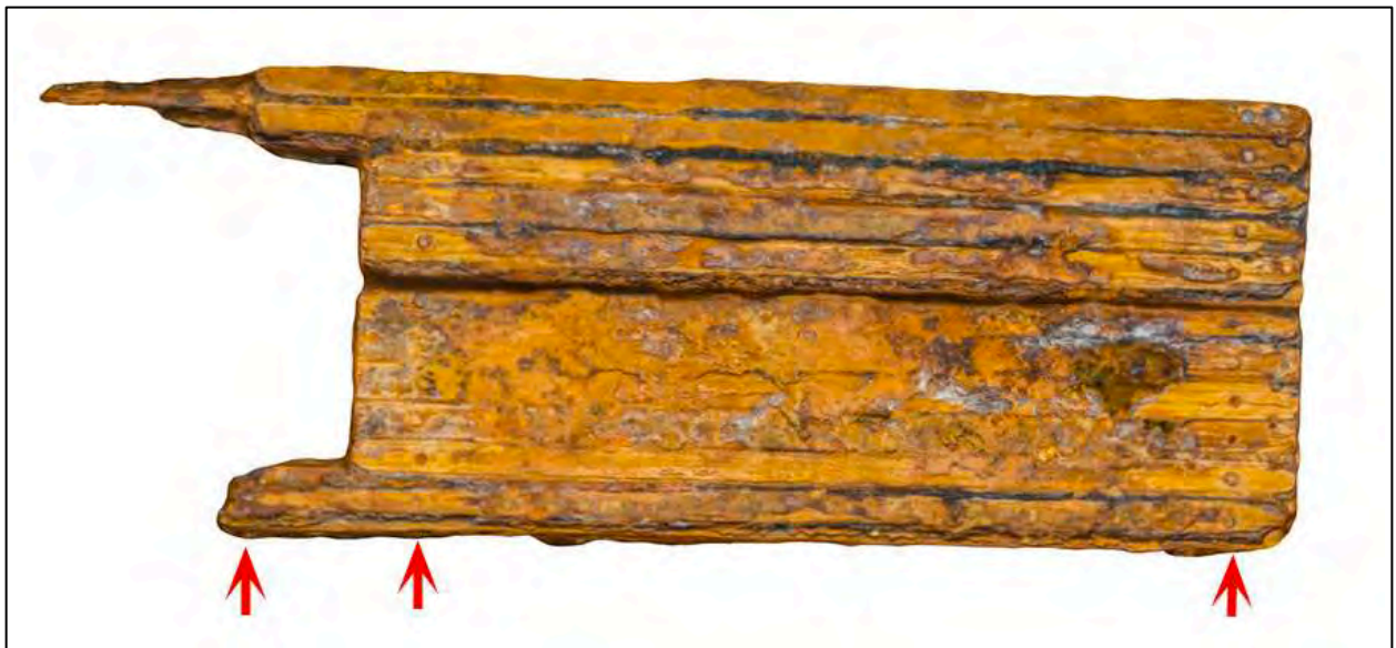
Figure 6-525. Orthomosaic of gunport (Lift WC-7) from West Casemate. At left is the 27-inch wide as-built cut-out for the cast iron gunport. The base of the casemate is at far right. It will be found to be the only gunport on the entire length of the West Casemate. Center arrow marks line of fasteners just to the right of the gunport that is found only below the gunport. The two other arrows point to line of fasteners that go completely across the casemate.
