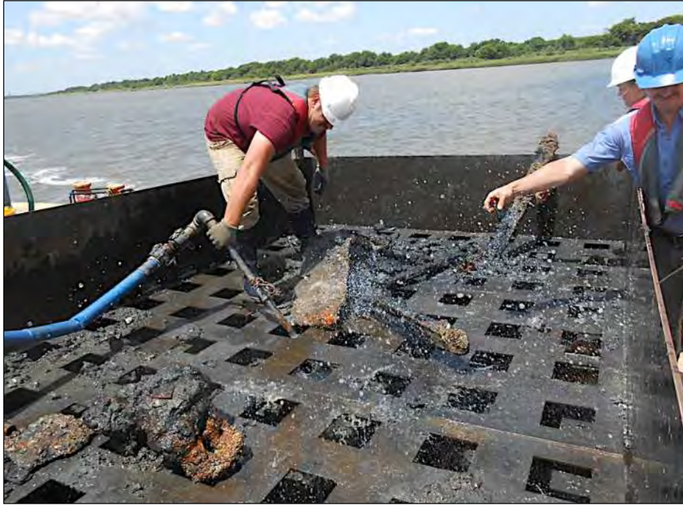
Figure 6-106. Initial processing of a clamshell grab. Over-built, the screen was difficult to access, affected processing efficiency, and raised safety concerns.
