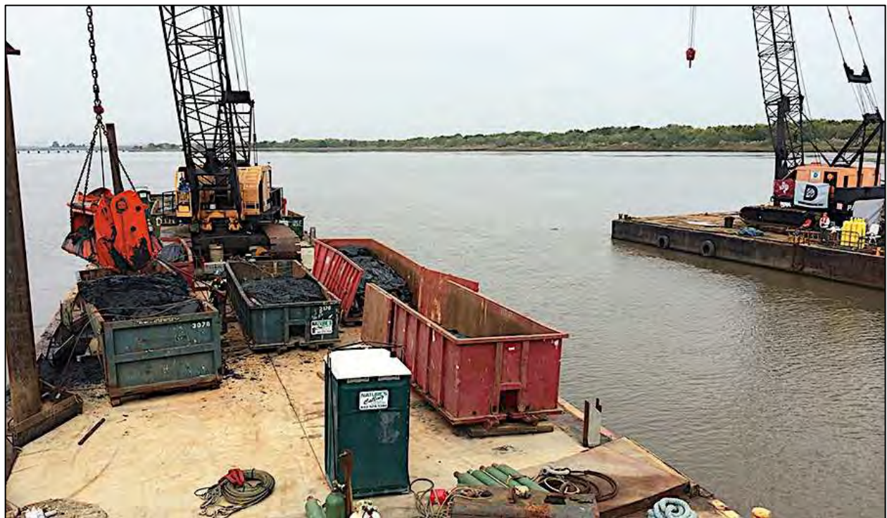
Figure 7-12. Clamshell filling containers with bottom sediments to keep the artifacts in place and enable the containers to sink immediately. Dive barge on the right was employed to send divers for burial verification.
