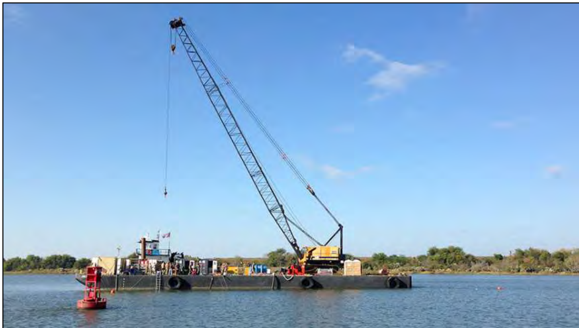
Figure 3-14. Barge on site with lift crane. Note the small orange West (left) and East (right) Casemate mooring balls that were employed to align the barge on the northern side of the site. Crane body is directly opposite the recovery section.
