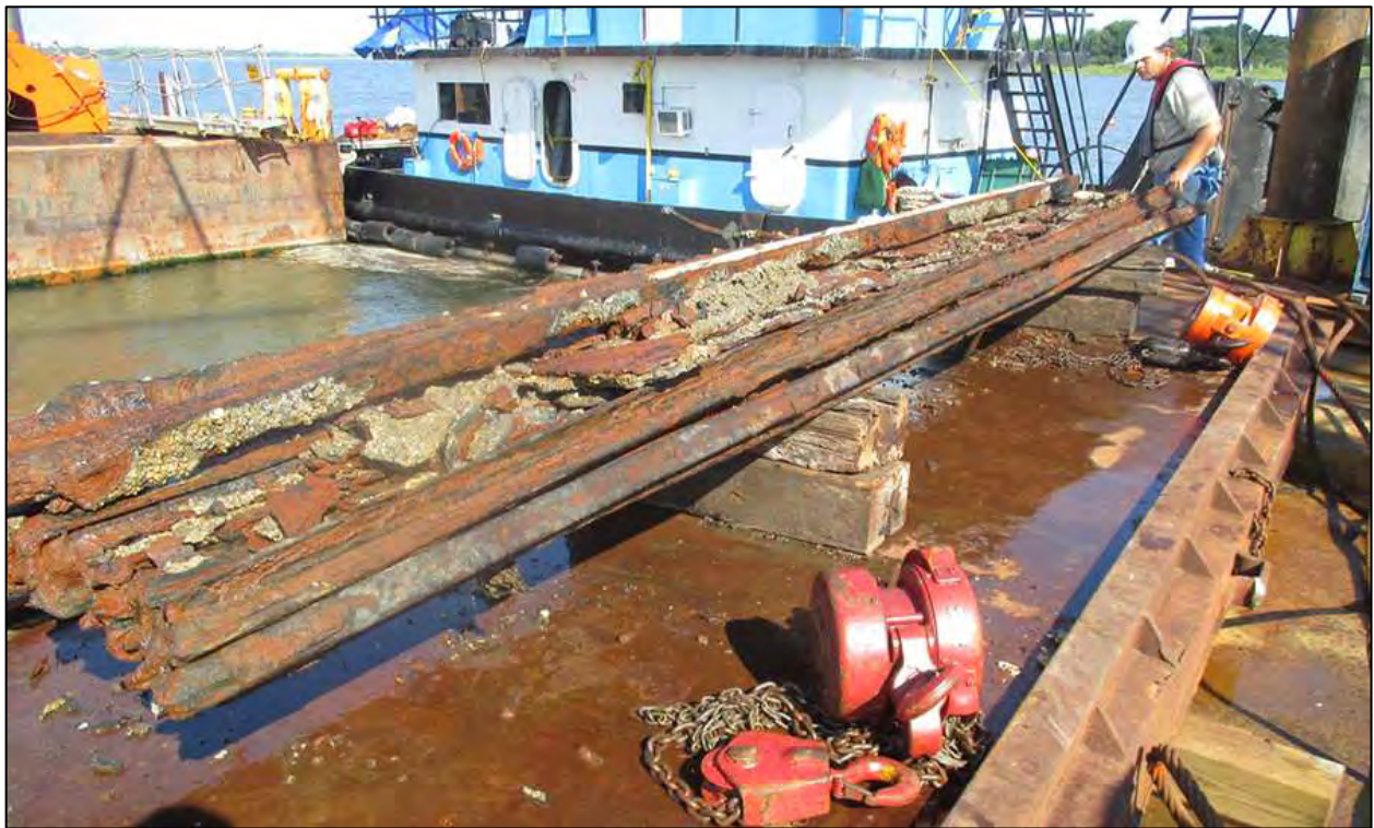
Figure 6-75. The fifth section recovered, located on the southern edge of the main casemate section, was detached with the rail separator. With no wood backing, the 24-foot long rails collapsed in on themselves when being raised.
