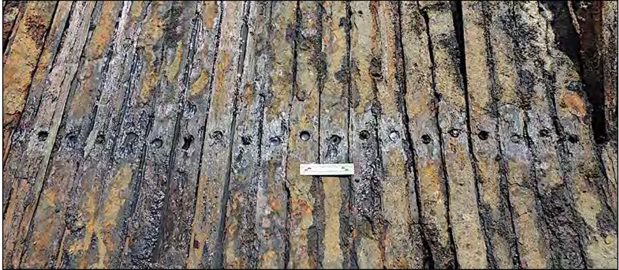
Figure 6-524. Bolts were used to secure the inverted rails to the 8-inch oak and 12-inch pine timbers, the bolts placed through a hole drilled through the center of the inverted rail.
