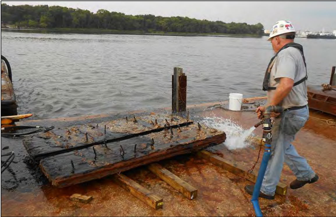
Figure 6-76. The sixth section recovered from the East Casemate. It has been separated into two sections on deck and is being readied for banding and subsequent transportation. The visible spikes are the location of the (now mostly non-extant) original wood backing.
