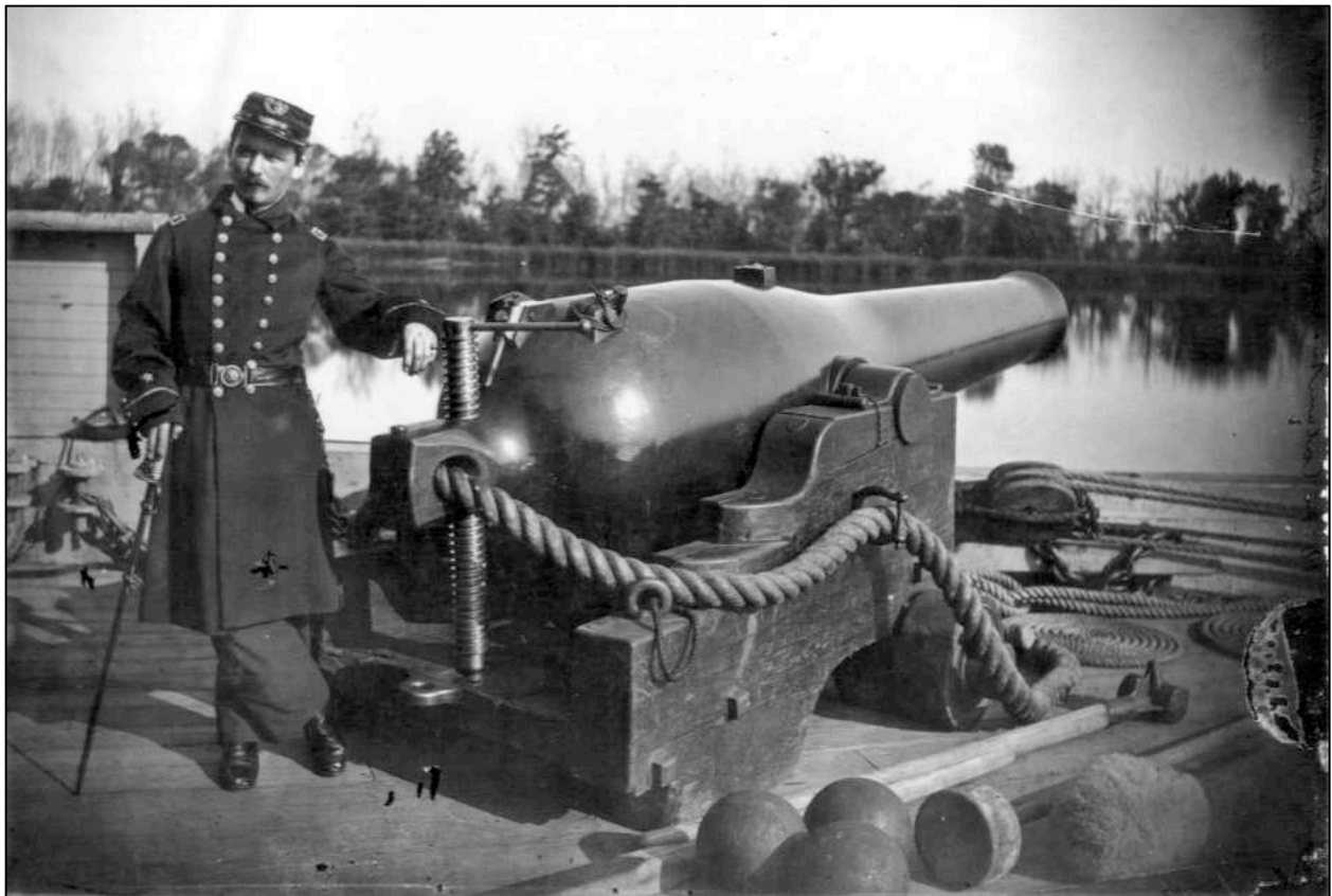
Figure 6-271. Dahlgren cannon on a Marsilly carriage on the USS Hunchback (U.S. National Archives Photo No. 111-B-2016, Brady Collection).
