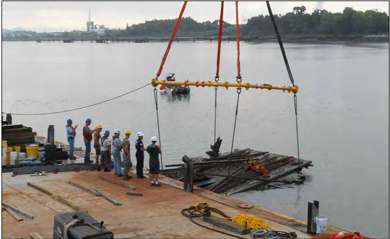
Figure 6-79. Similar to the first lift attempt, after the casemate broke the surface, it was held stationary to enable engineers to check the rigging and general load for safety. Remaining in this position for several minutes, it was thought to still be too unstable to lift free of the water, as there was no wood backing on the northern half. It was lowered back to the riverbed and de-rigged. As discussed below, it would be recovered in 2017 employing a different lifting method.
