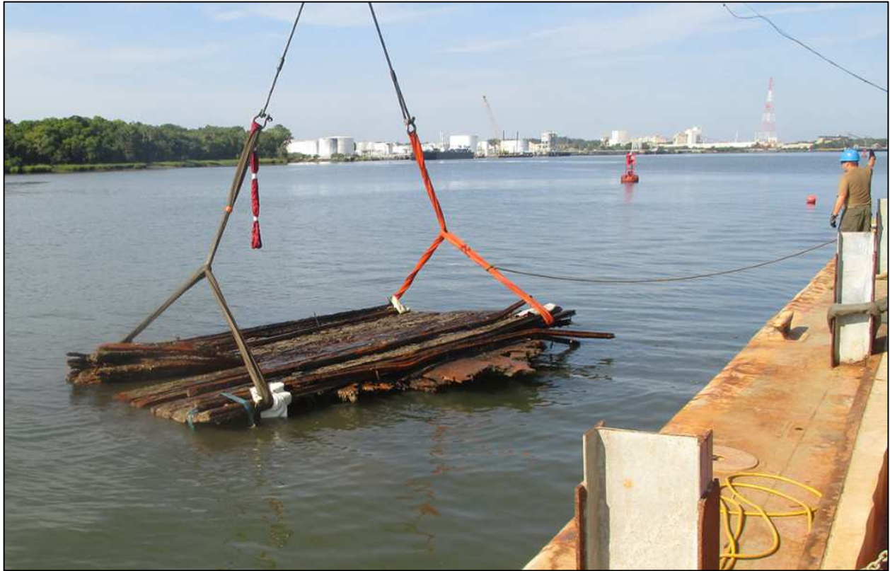
Figure 6-77. The first attempt at raising the large, intact East Casemate section in 2015. Immediately after this photograph was taken, the sling at right slipped off the rail ends and the entire section fell back to the riverbed.
