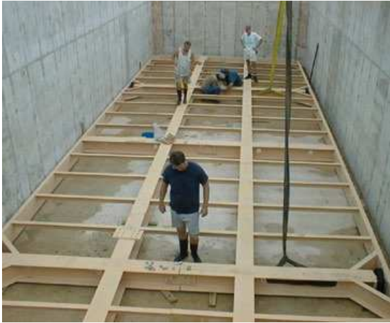
Laboratory assistants Dan Walker, Jim Jobling, Peter Fix, and Peter Hitchcock bolt the two halves of the frame together.
