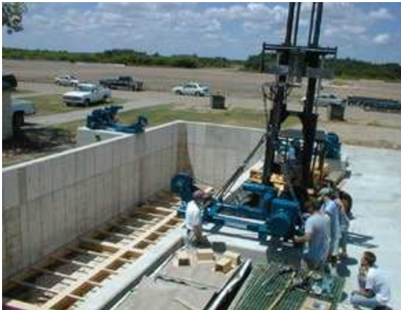
Installing one of four winches
