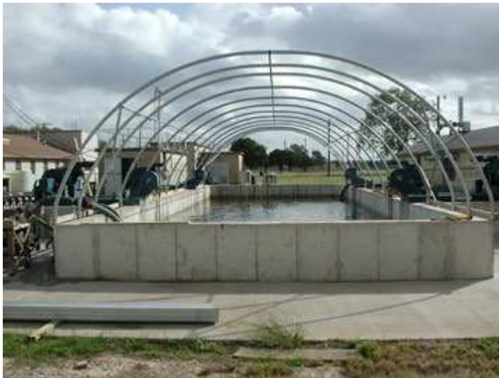
The roof was constructed from a modified greenhouse kit.
