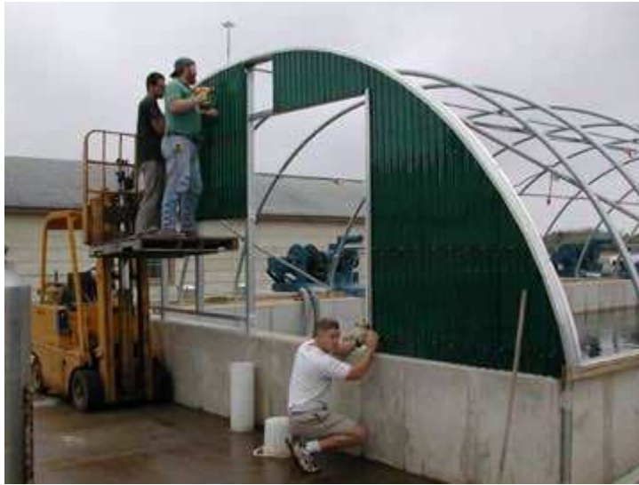
Corrugated fiberglass panelling was used to construct the ends of the structure.
