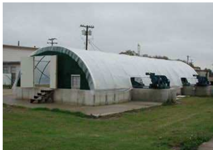
View of the newly built cover built over the treatment pool. The roof was constructed from a modified greenhouse kit.
