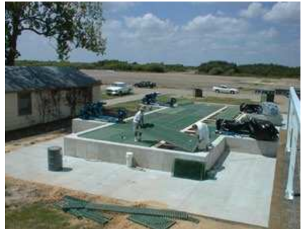
Installing the fiberglass grating on the lift
