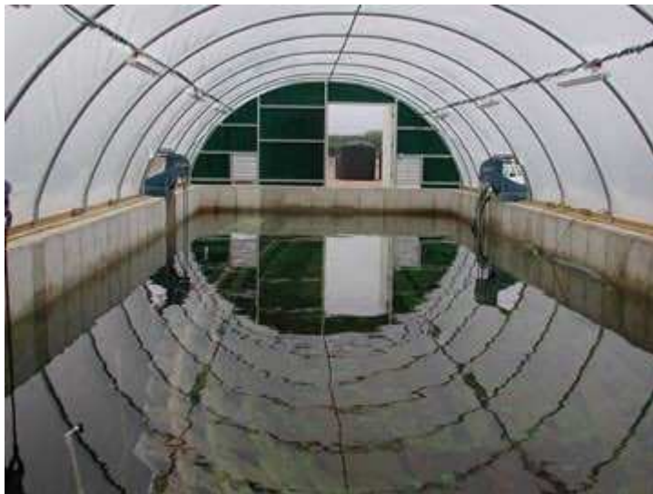
The frame was covered with two layers of clear plastic that are inflated to provide an insulating barrier. A third layer of black plastic will be used to protect the ship from sunlight and to retain heat, as well as to retard algae growth.
